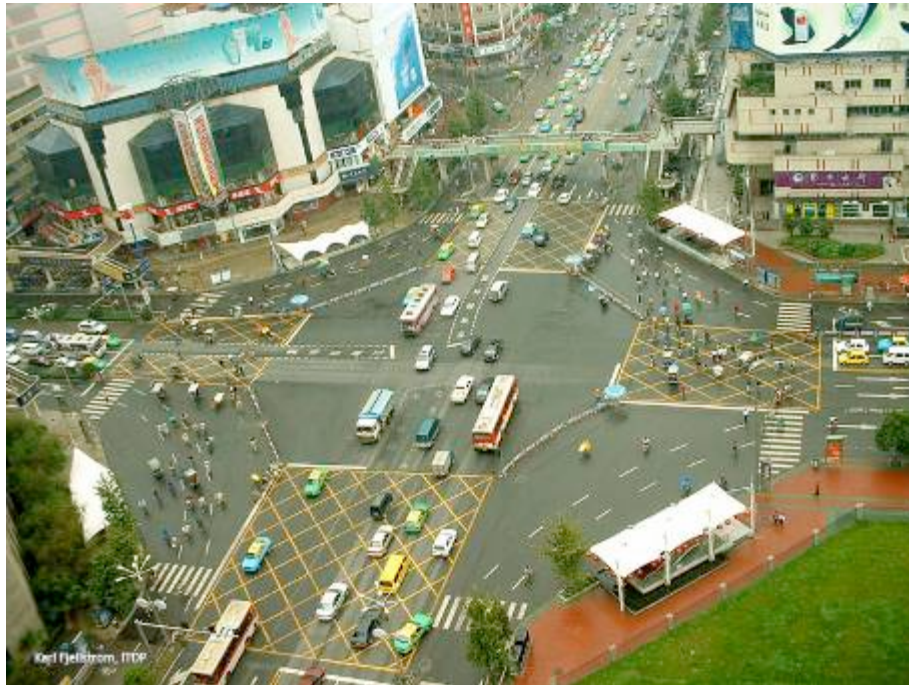
Figure 16. Cyclists at Traffic Intersections in Chengdu, PRC
