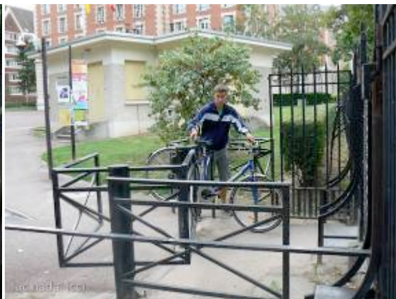
Figure 19. Motorcycle-Proof but Pedestrian, bicycle, and Wheelchair-Accessible Gate in Paris, France Photo: Luc Nadal
