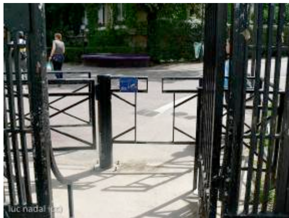
Figure 19. Motorcycle-Proof but Pedestrian, bicycle, and Wheelchair-Accessible Gate in Paris, France Photo: Luc Nadal
