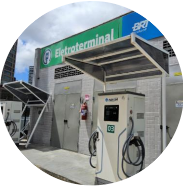
Construction of 2 new charging terminals
