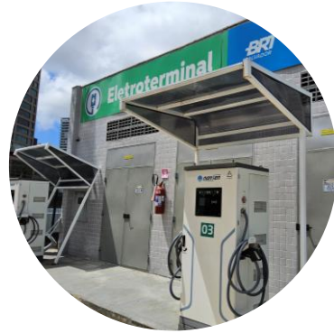
Construction of 2 new charging terminals
