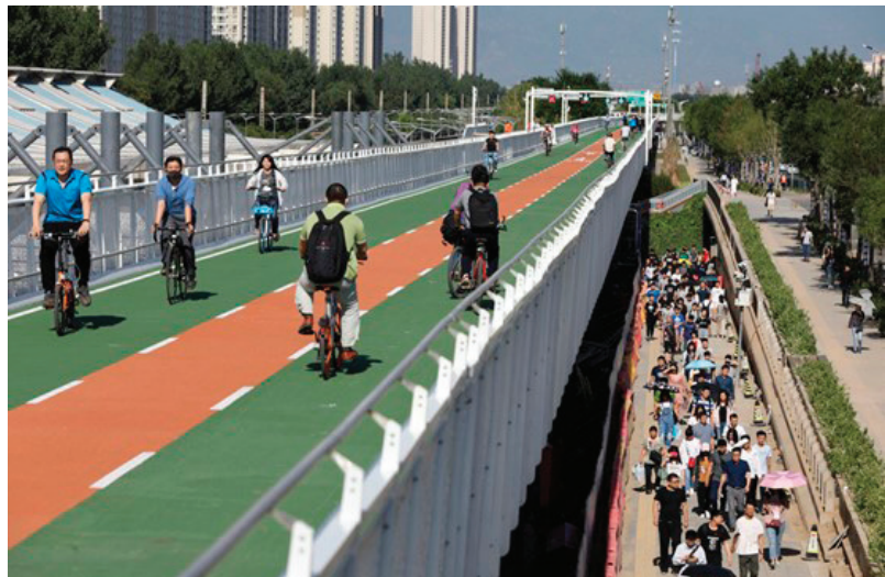
Cities in China have been investing in innovative cycling infrastructure, like this elevated greenway. Photo: ITDP China
