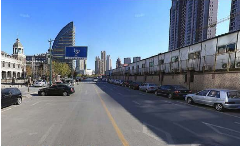
Before and After look of Shuige Road
