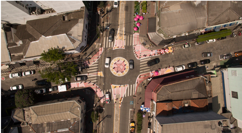
In the Santana neighborhood of São Paulo, Brazil, a few on-street parking spaces were repurposed to daylight a major intersection, improving safety and comfort. SOURCE: Tomaz Cavallieri, WRI Brasil
