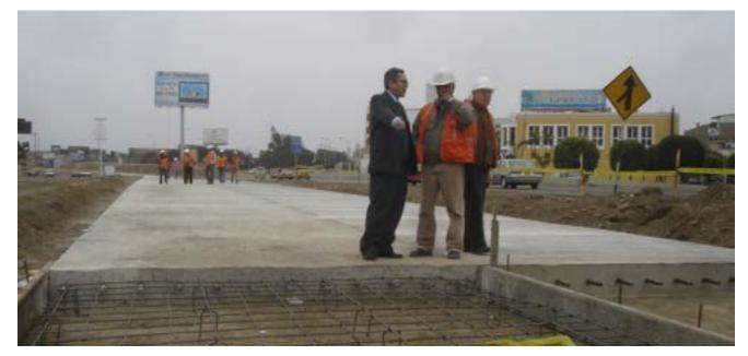
Reinforced concrete pavement under construction in Lima, Perú. **CREDIT:** Gerhard Menckhoff • **Continuously Reinforced Concrete Pavement:** Continuous slab reinforcement can add additional pavement strength and might be considered under certain design conditions.
