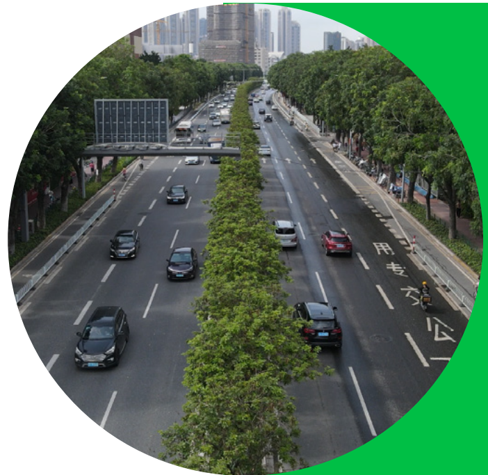
Huadi Avenue North in Guangzhou, China is a complete street that incorporates protected bicycle lanes. Source: ITDP China
