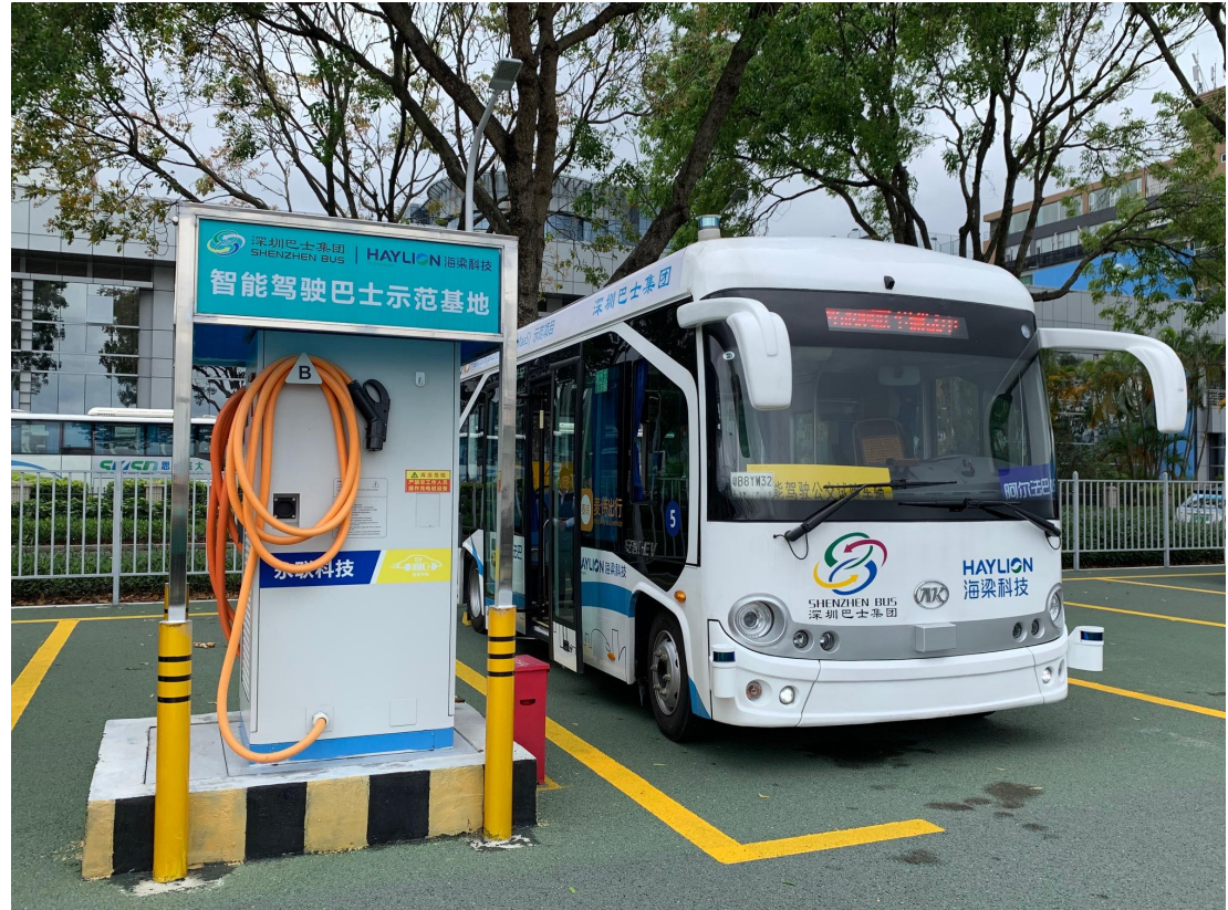
An electric bus and plug-in charger in Shenzhen, China. SOURCE: ITDP China.
