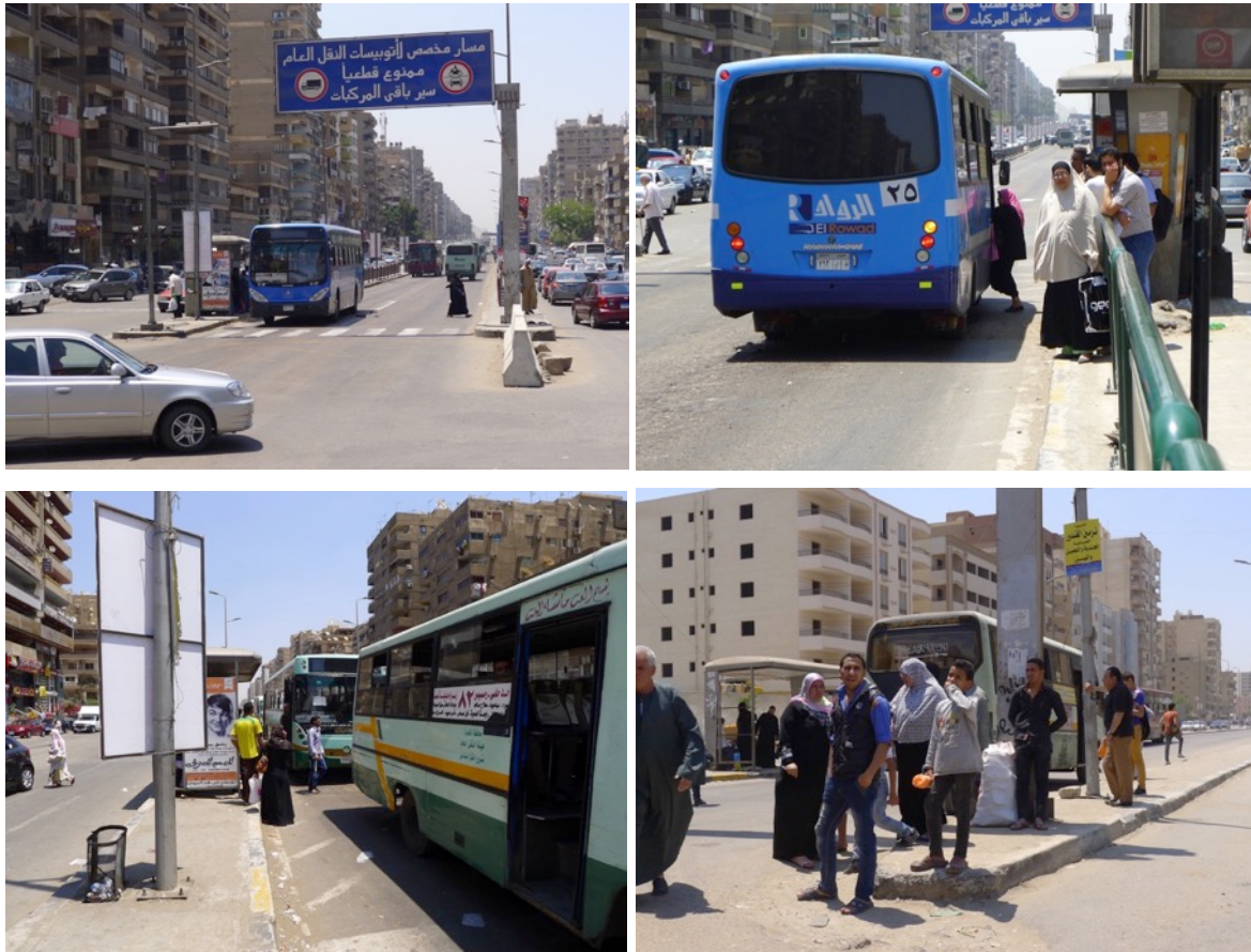
Figure 10: The Mostafa El Nahaas busway in Nasr City offers dedicated, median-aligned bus lanes (top left), but lacks other essential features of BRT, including level boarding and off-board fare collection. Passengers struggle to board buses with multiple steps (top right). Shelters are poorly designed (bottom left) or entirely absent (bottom right).
