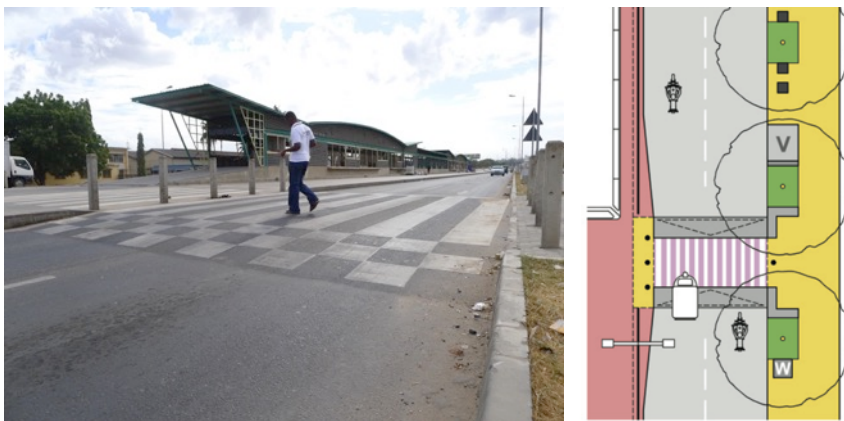
Figure 39: Access to midblock BRT stations should be provided through tabletop crossings at the same level as the adjacent footpath to improve accessibility.
