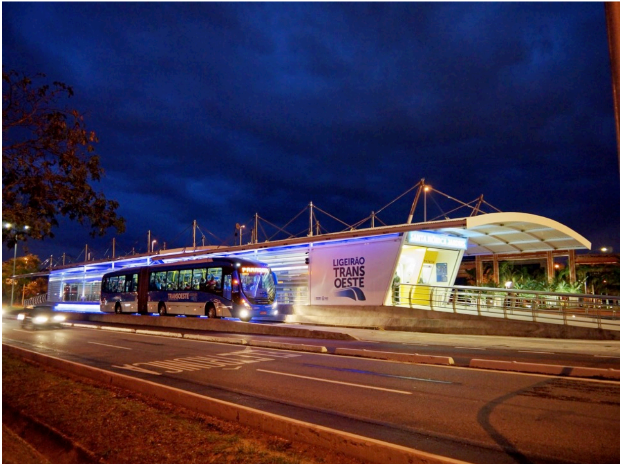
Figure 30: Iconic station designs, such as those in Rio de Janeiro’s TransOeste corridor, can raise the profile of the BRT system.
