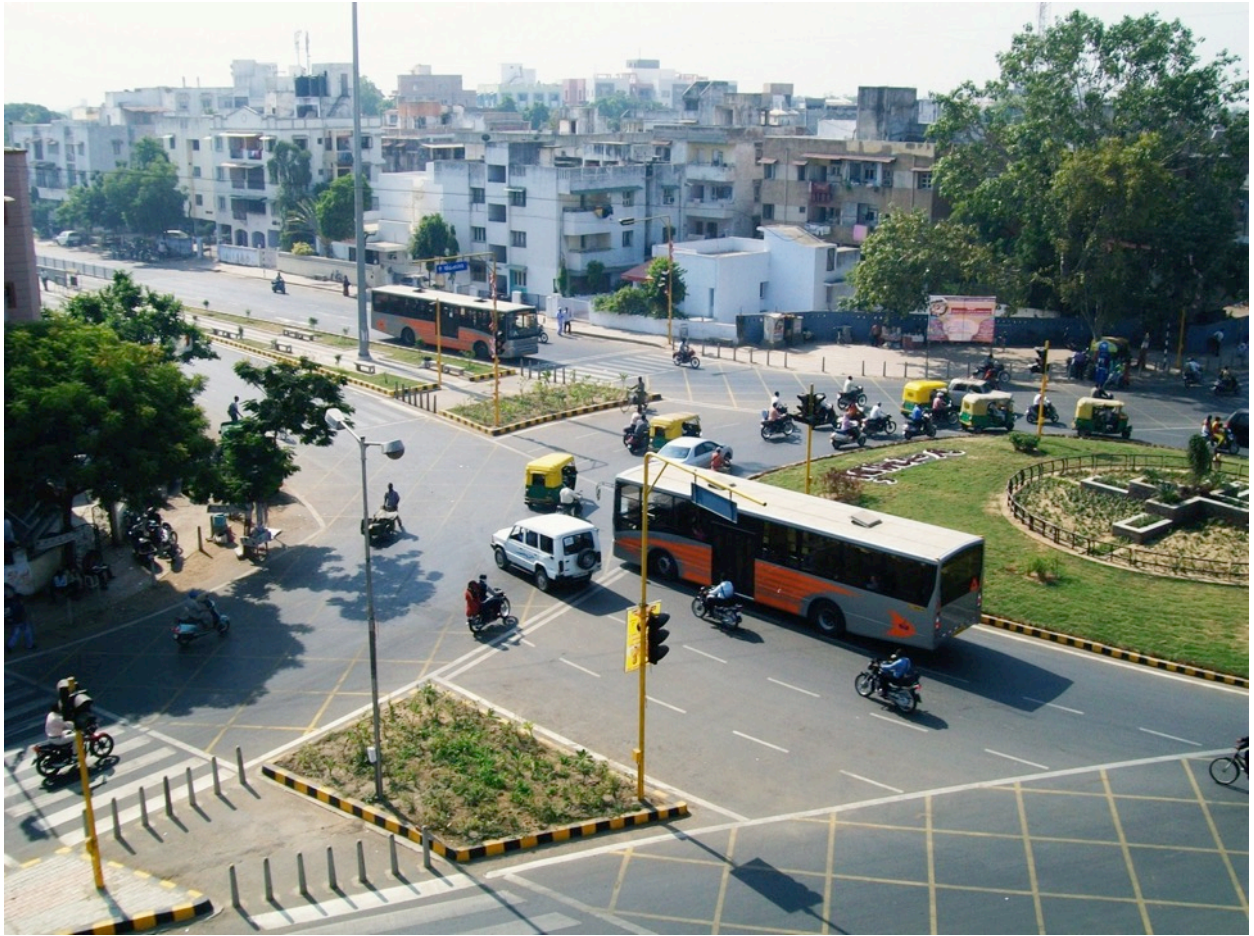
Figure 36: Two-phase squareabout intersection in Ahmedabad, India.
