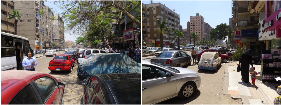
Figure 43: Unorganised on-street parking occupies a large amount of road space and compromises pedestrian access. Defined parking areas and performance-based pricing can help improve
